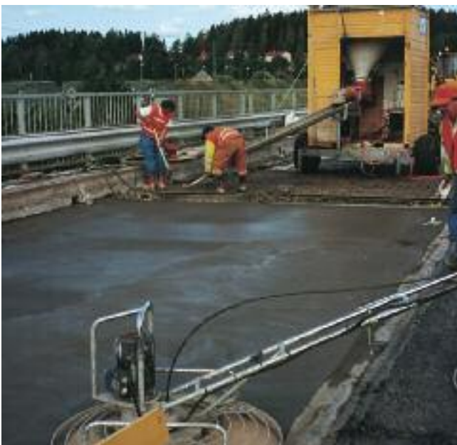
Bro under reparation
